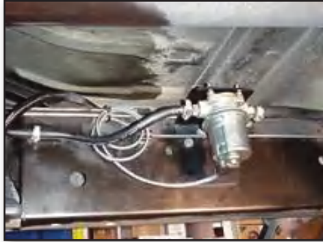
The finished installation.
