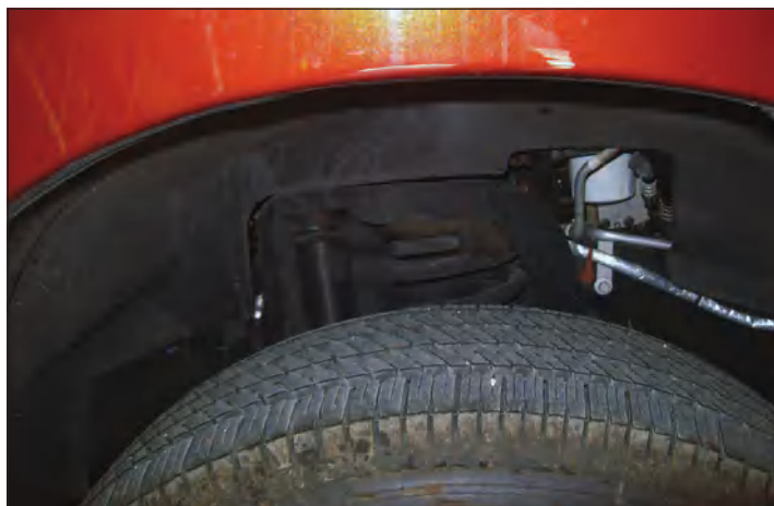
Initial view above right front tire with turbocharger covered by plastic inner fender. The shock absorber/ coil spring tower can be seen, but not the turbocharger.
