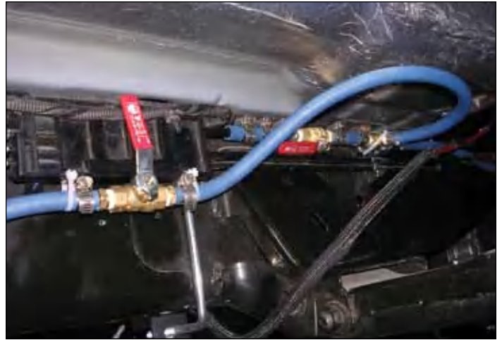
Stock valve is open, FASS valve is closed.
