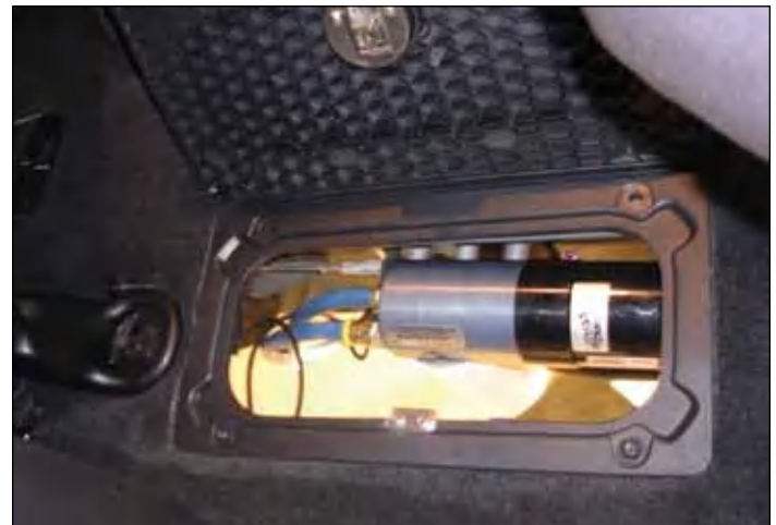
From above, a picture of the FASS unit that I installed on the outside of the driver's side frame rail.
