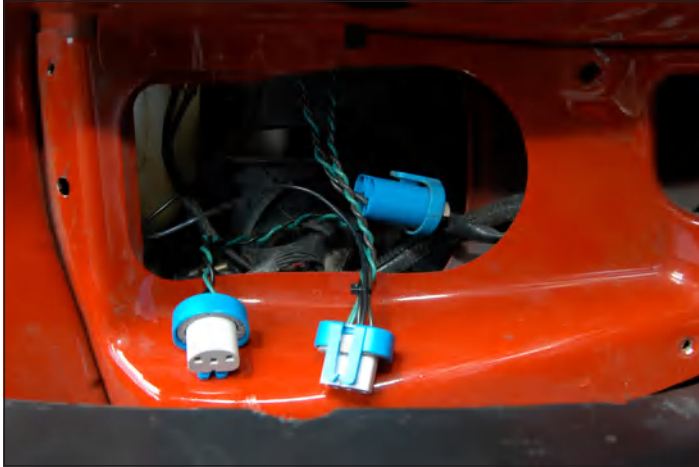
The Brite Box adapter harness installed.
