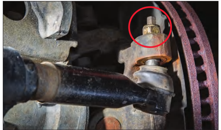
Figure 8: Dropping the old Y-type tie rod from the driver-side steering knuckle. The nut in this photograph (circled) is only partially removed.
